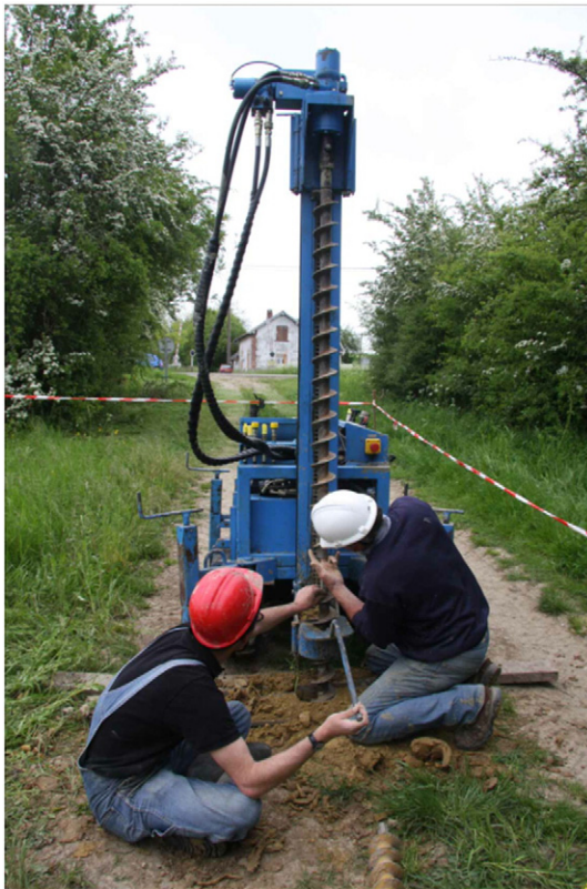
Fig. 4. Photography of the helical auger used for the geotechnical investigation.
